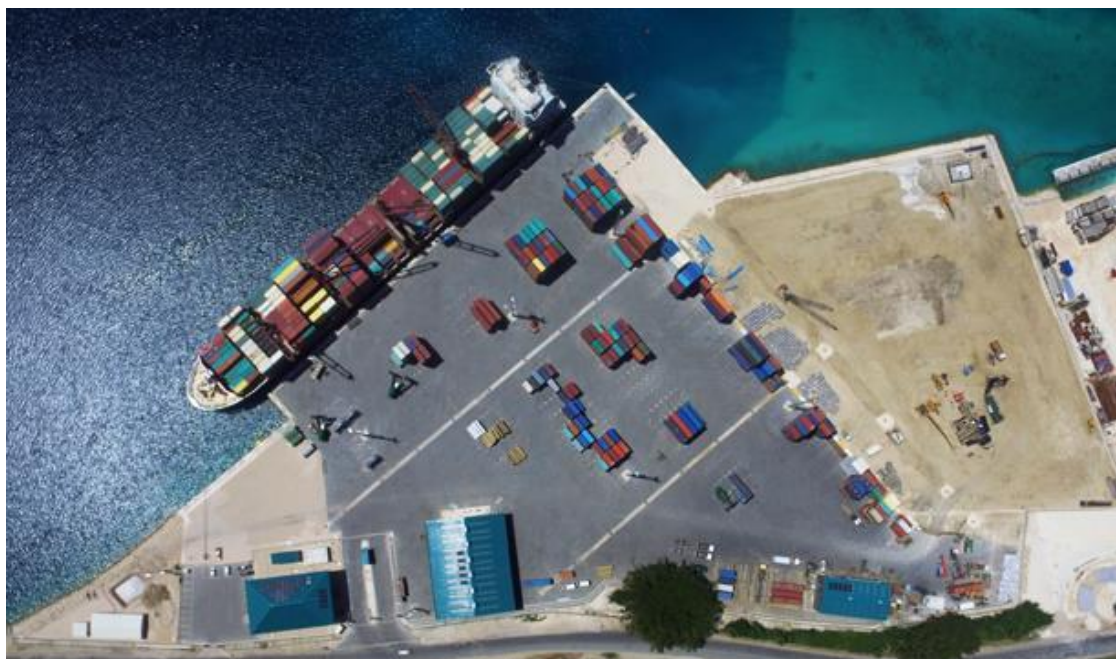
Figure 21 - Lapetasi Wharf and Terminal Port Vila, Vanuatu 2018 (VPMU, 2018)
