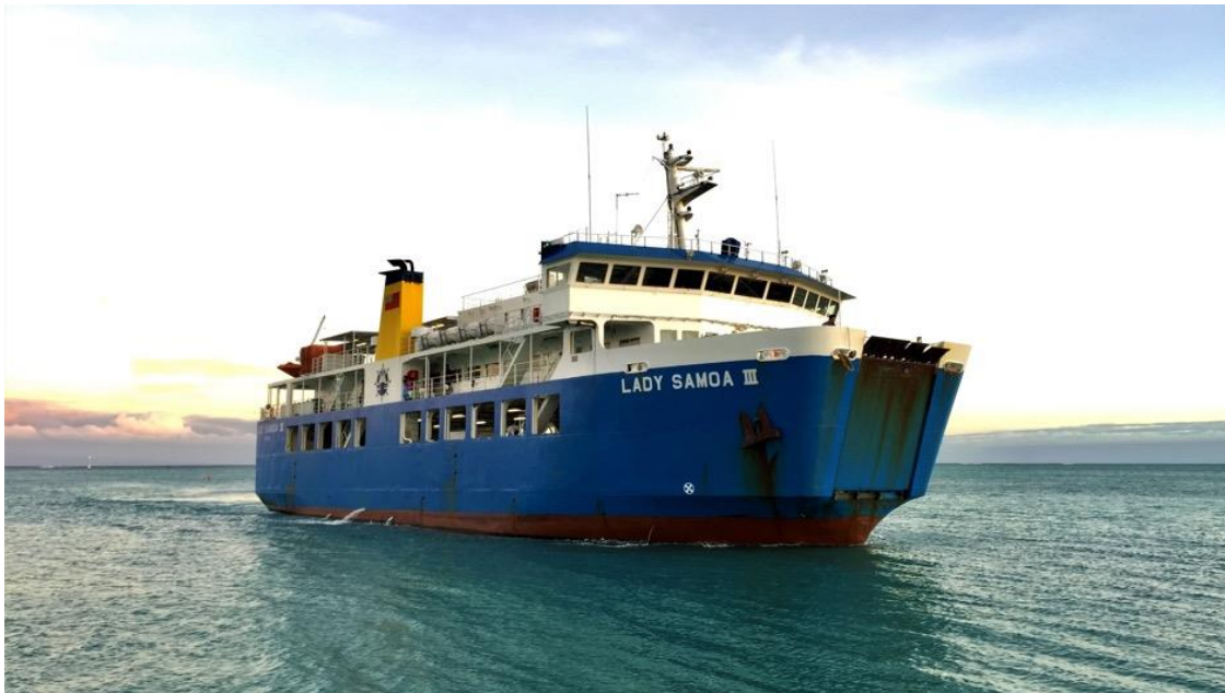
Figure 23 - Typical Purpose-Built Passenger Ferry Samoa 2016 (AMSTEC Pty Ltd)
