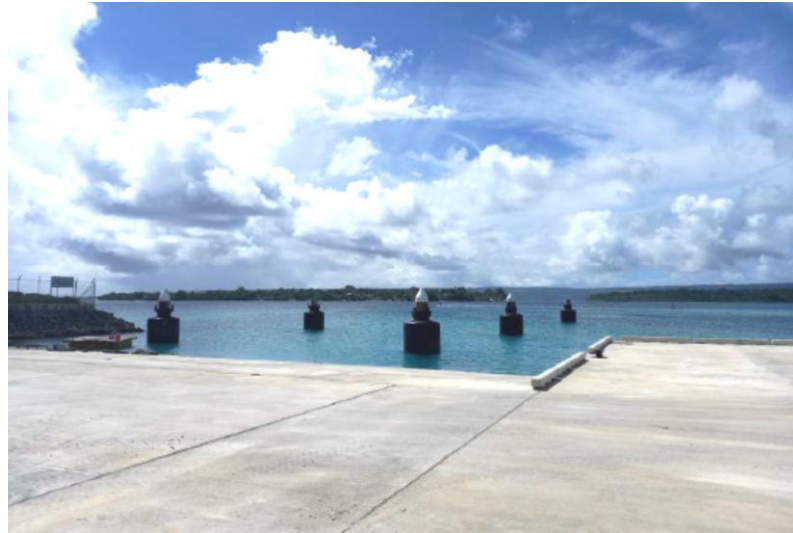
Figure 3 - Mooring piles and floating fenders have been completed.
