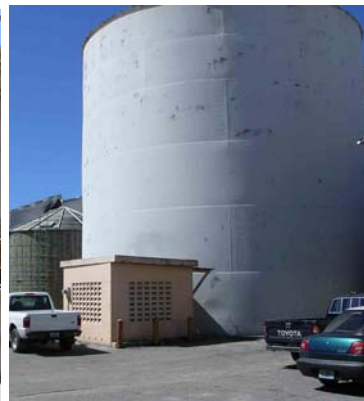
Crude Oil Storage 3000 tons
