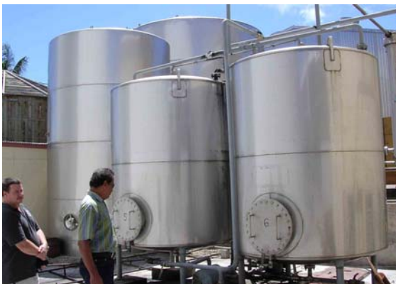
Refined Oil Storage
