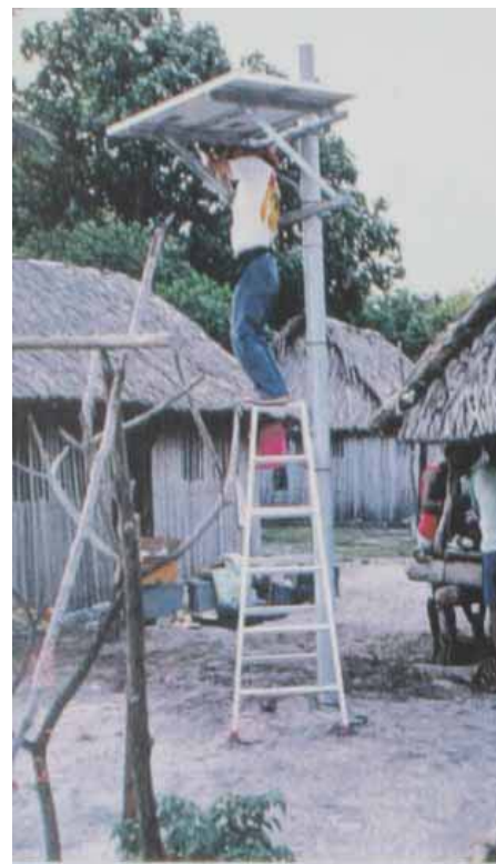
Figure 4-4 - Household panel Installation
