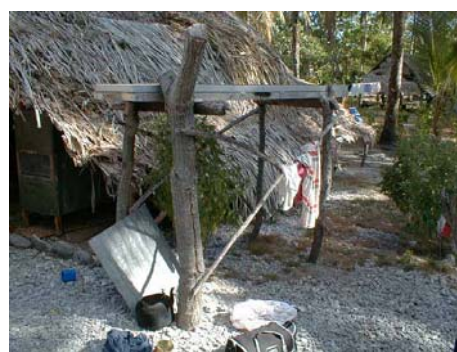
Figure 4-2 - Private solar installation
