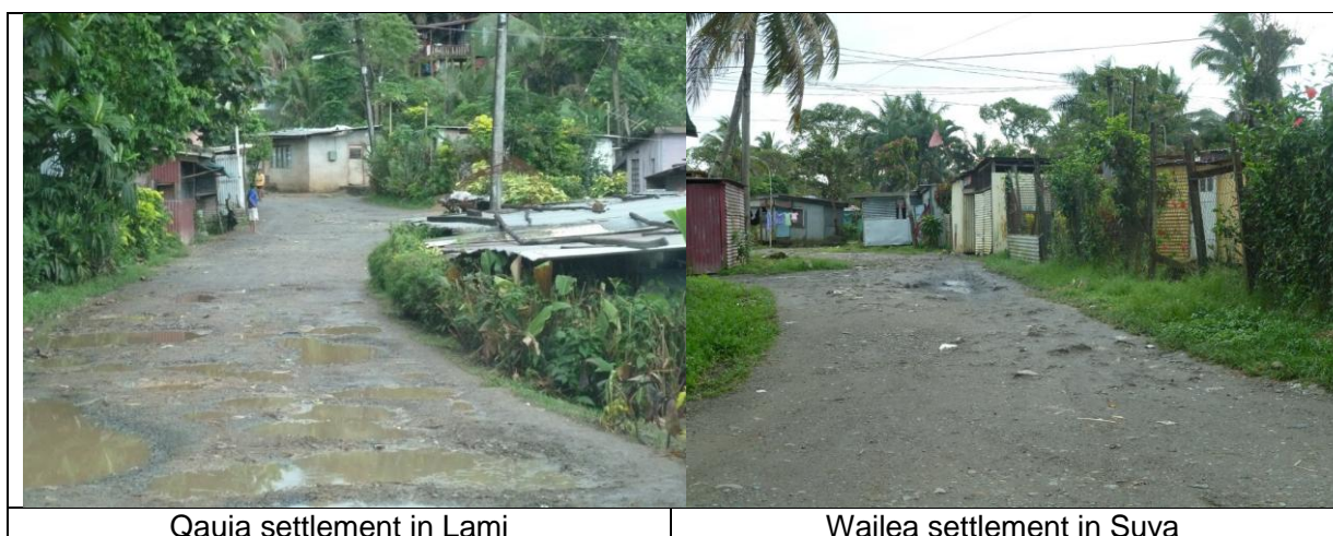
Figure 5.2: Existing Road Infrastructure Conditions in Informal Settlements
