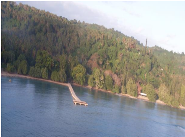
Figure 2.0 Domestic Ships jetty (outer-island)
